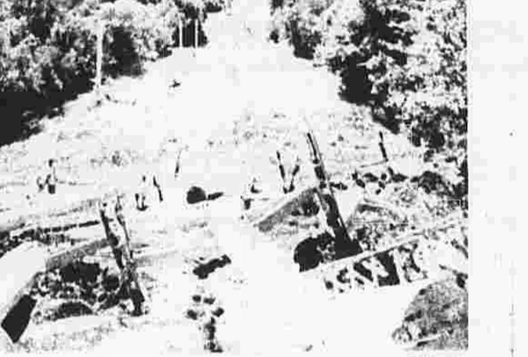
After August, winter double to a four-person quad chairlift. The old towers, in foreground, will be extended and put back into place next week.
